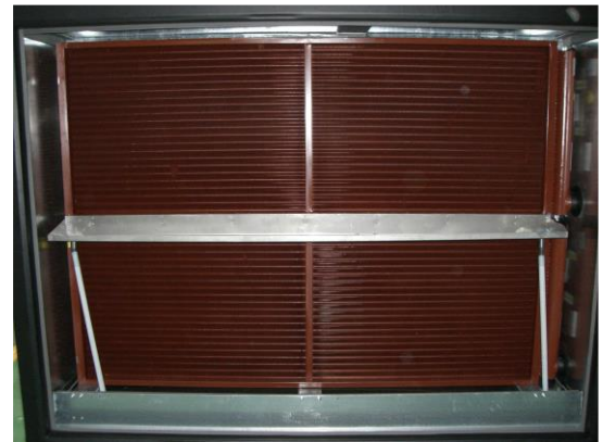
Figure 5: Stacked Coil
