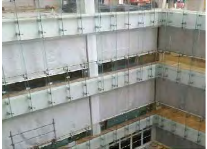
| Atrium Smoke Baffles used in conjunction with smoke venting/exhaust systems
