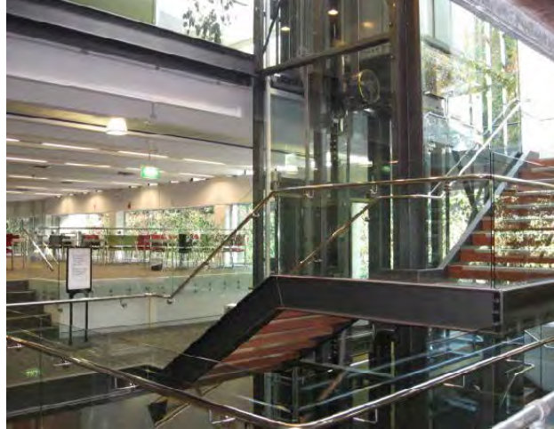
| University Fire & Smoke Compartmentation
