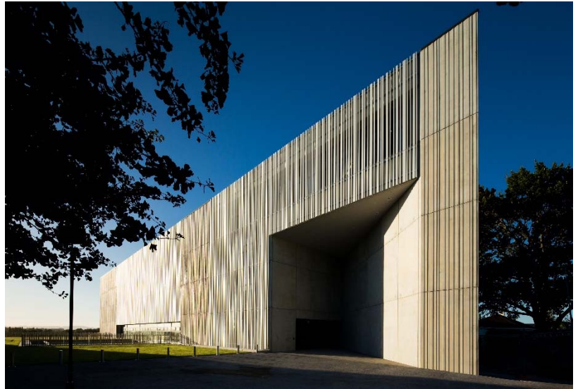
Clip-on cladding with vertical rebates – University of Waikato Law Building
