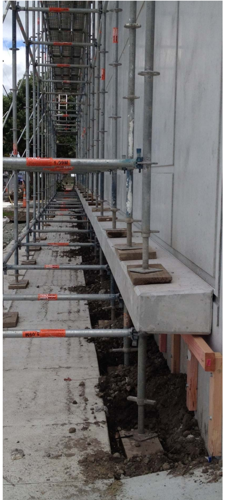
Litecrete sills being attached to Litecrete wall panels—Countdown Orewa
