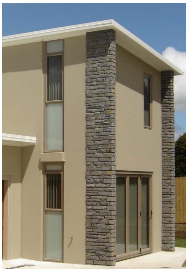
Stone veneer adhesive-fixed to Litecrete panels
