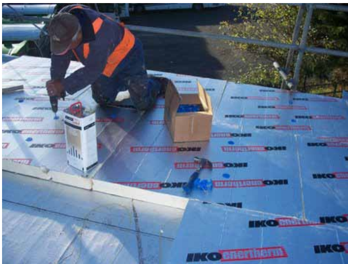
Insulation set out on plywood
