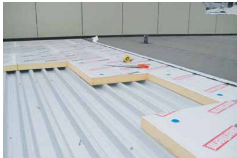
Insulation fixing on metal roofing
