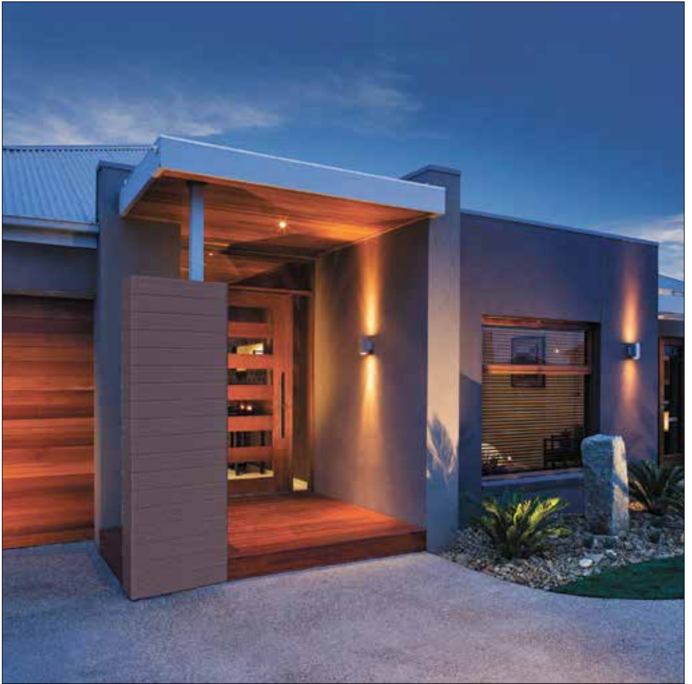
An example of a home built with Hebel.
