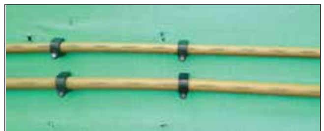
Fig. 3.2 – Installed piping services prior to the installation of Hebel PowerPanel XL
