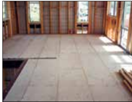
Fig 1.2 Residential Suspended First Floors
