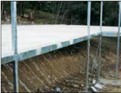
Fig 1.1 Residential Suspended Ground Floors
