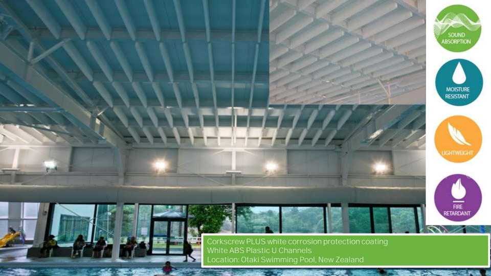
Vertical baffles with no bracing profile.
