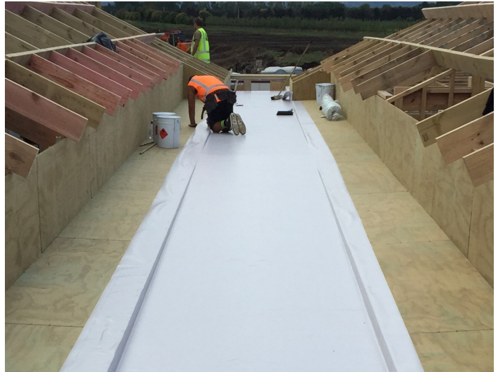
Rooflogic Fibertite SM being adhered to plywood gutters with RL 190E
