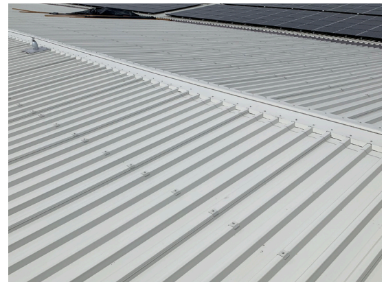
Topdeck T installed on a Rooflogic MSR System.
