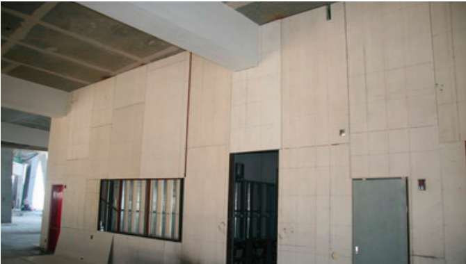
Shenzhen Futian Library: In production
