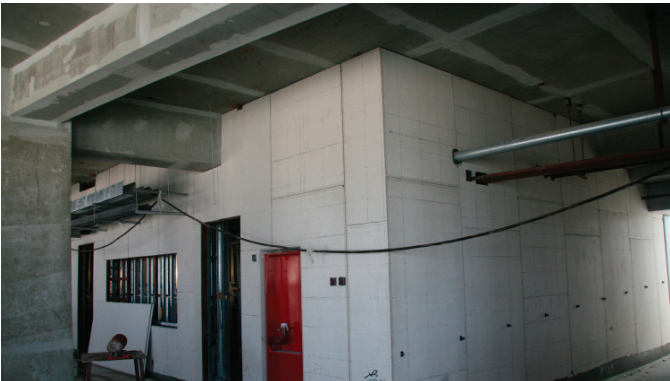
National Stadium(The Bird's Nest) - In Production
