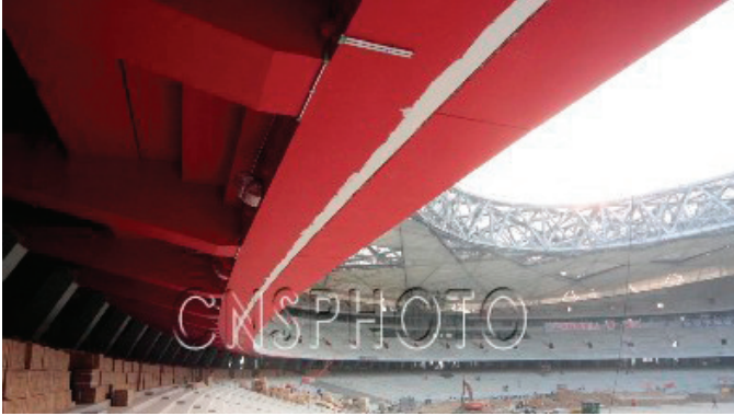
National Stadium(The Bird's Nest) - In Production
