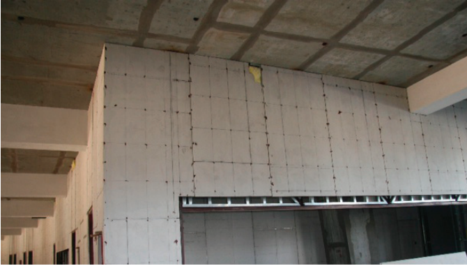
Shenzhen Futian Library: In production
