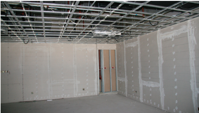
National Stadium(The Bird's Nest) - In Production
