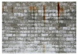
Figure 8Acid burn on concrete masonry block
