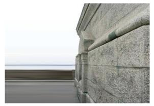
**Fig 9** Copper stains on face block work
