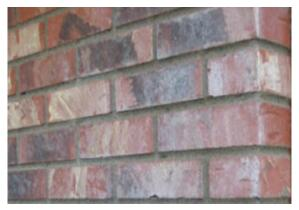
Figure 7Calcium carbonate on face block work
