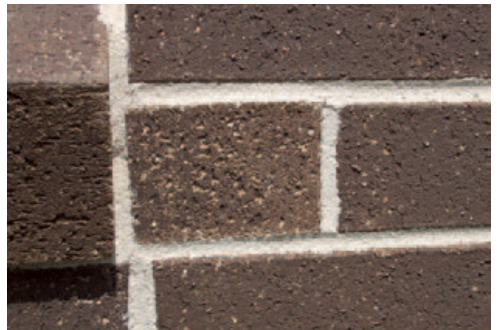
Damage to ironed mortar joint
