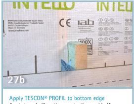
Apply tape half on the penetration and half on INTELLO®. Cut at 45° and 3 mm away from the corner of the penetration and fold it up as shown.
