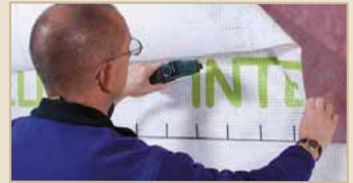
Fig. 86. Taping overlaps
