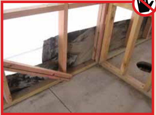
Fig. 79. Bitumen membrane outdoors
