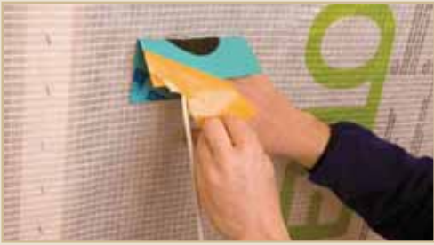
Fig. 90. ROFLEX pipe grommet fixed with TESCON VANA
