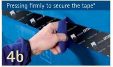
Press firmly to secure the tape, ensuring there is sufficient pressure, for example using a pro clima PRESSFIX to do the job effectively and to protect your hands.
