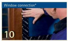
Seal the wall protection membranes to the joinery using the TESCON EXTORA tape to ensure the connection is windproof and weathertight.
