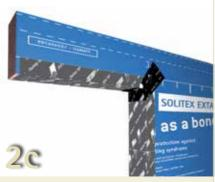
Cut and apply a small strip 100 mm x 150 mm to reinforce the corner.
