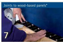
To create weathertight joints between wall protection membranes and smooth, non-mineral surfaces such as wood-based panels or planed wood, place TESCON EXTORA centrally over the joint, unroll and stick down over the joint.
