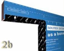
Cut and fit a length of TESCON EXTORA to be filled 100 mm down the jambs and 100 mm along the lintel.
