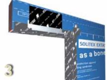
Once both studs are installed, cut the TESCON EXTORA tape for the head flashing to suit. The tape needs to extend the entire length of the flashing. Note: Shortened head flashing shown for clarity
