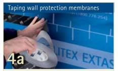
Place TESCON EXTORA centrally over the overlap (minimum 75 mm horizontally and 150 mm vertically), unroll and press down over the joint.
