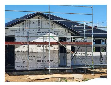
IBS RigidRAP®-XT comprises of an 8mm thick, moisture-resistant, oriented strand board (OSB3) panel with a synthetic wall underlay adhered to the outer face and a 10mm thermal break on the inside face suitable for use as a wall bracing element, structural rigid air barrier. Designed primarily for steel frame construction but can also be used with timber frame construction.
