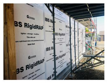
IBS RigidRAP® comprises of an 8mm thick, moisture-resistant, oriented strand board (OSB3) panel with a synthetic wall underlay adhered to the outer face, suitable for use as a wall bracing element, structural rigid air barrier.
