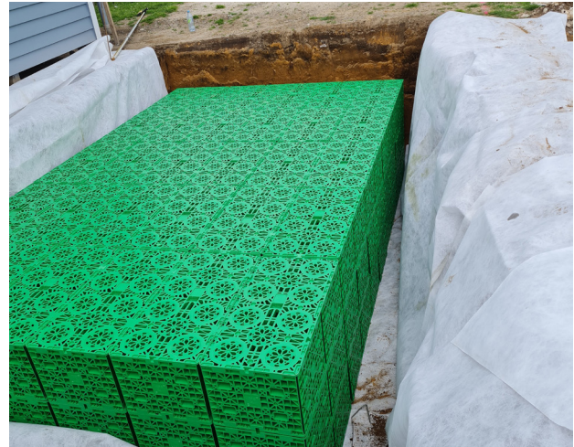
Wrapped StormCell Modules & Back-Filling
