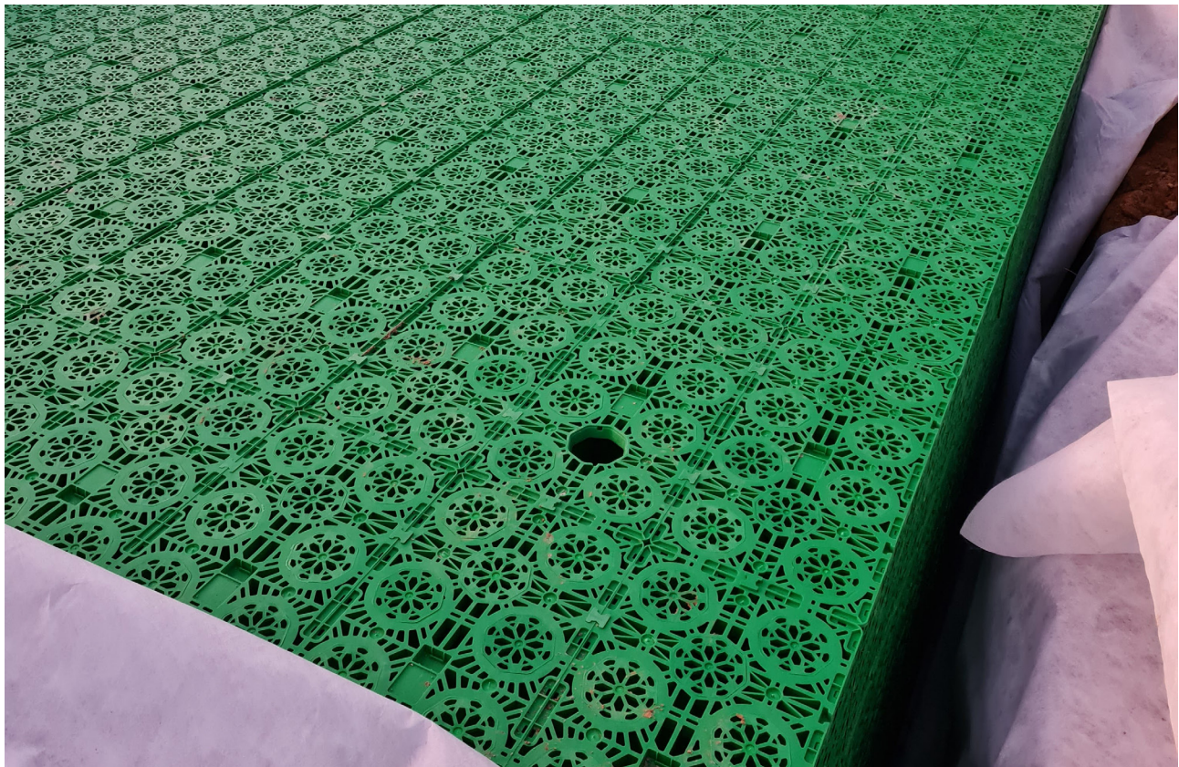
Completed StormCell System Construction
