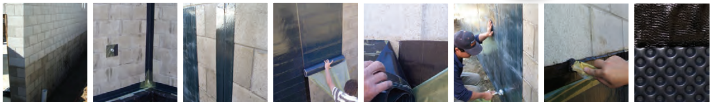
Wall area is primed before installation.
