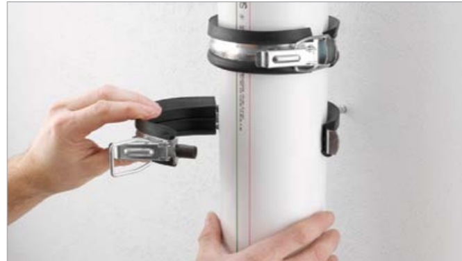
Fig. 7-2 Closing supporting clamp.
