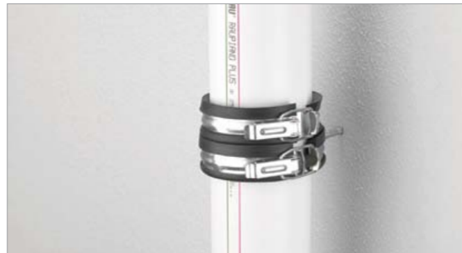
Fig. 7-3 Fully installed support bracket.
