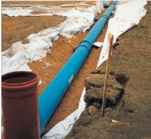
Illustration 10-32: Installing drainage in the playing field
