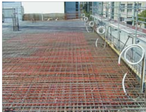
Illustration 9-2: Concrete core temperature control concreting section
