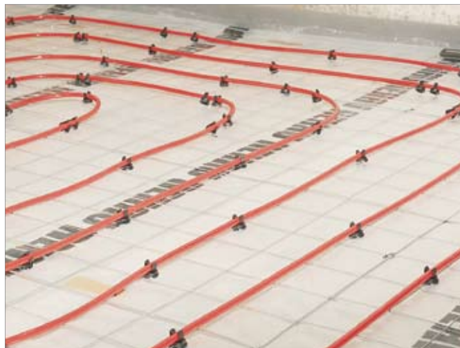
Illustration 4-46: REHAU pipe grid system
