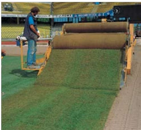
Illustration 10-33: Installing pitch
