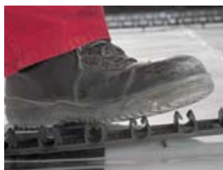
Illustration 4-42: Pressing REHAU RAUFIX rail into the floor
