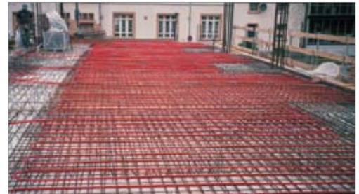
Illustration 9-4: REHAU BKT modules on pre-fabricated concrete parts
