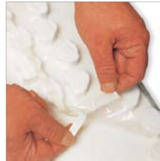
Illustration 6-2: Attaching the film base on the REHAU vario studded panel
