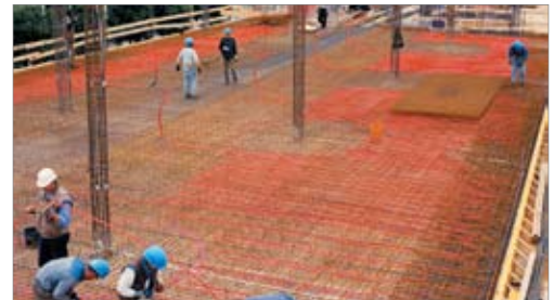
Illustration 9-5: REHAU concrete core temperature control installed on site
