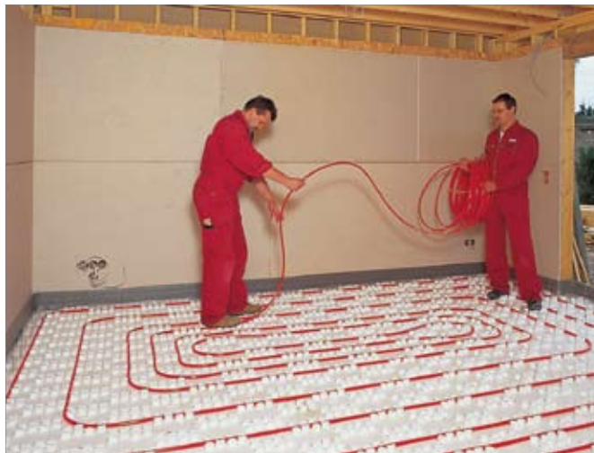
Illustration 4-26: Installing pipes on the REHAU vario studded panel
