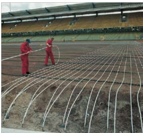
Illustration 10-35: Installing heating pipes
