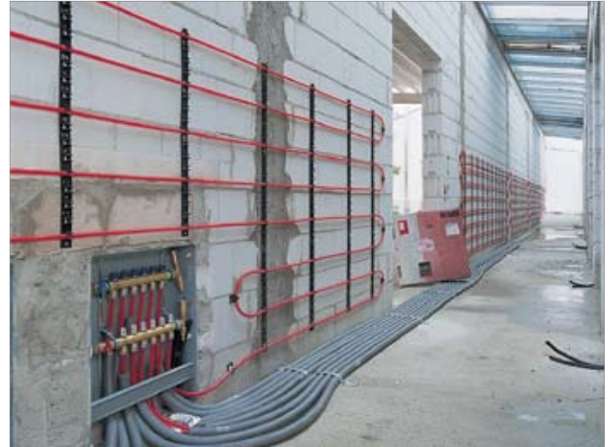
Illustration 5-10: REHAU wall heating/cooling with wet construction
