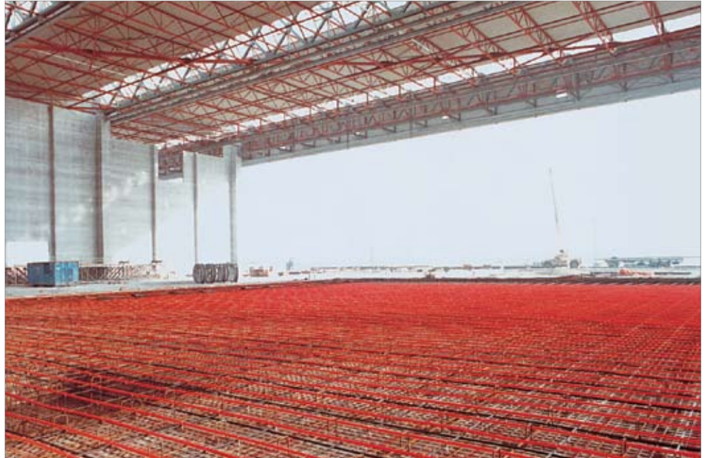
Illustration 10-1: Underfloor heating in an industrial hall
