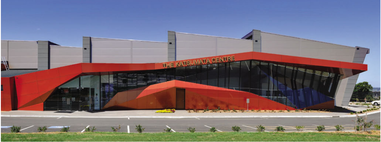
The Katsumata Centre, Geelong, Victoria, Australia.
