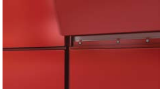
Subsequent cassettes hook into neighbour, next layer fixes into lower layer and neighbours.
