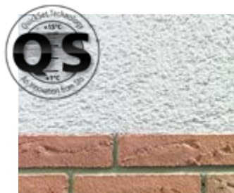
Intact facade with QS Technology
