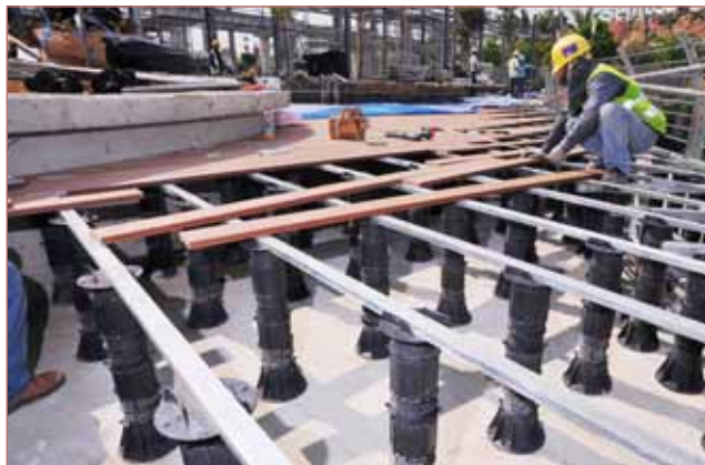
VersiJack® F provides stable support for installation of decking
