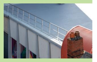
weldable Viking Enviroclad TPO membrane were installed with no end-laps as each roll extended the full width of the roof.
