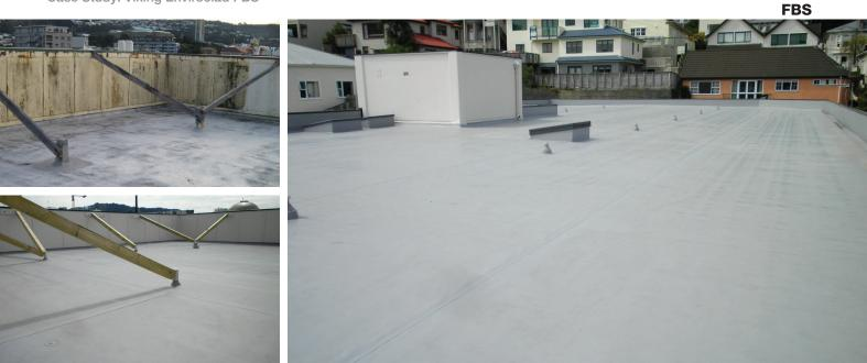
The Viking Approved Applicator then set about installing 1300m2 of Enviroclad F.B.S. with its 3.6m x 30.4m (109.8m2) rolls and F.A.S.T. adhesive system.
