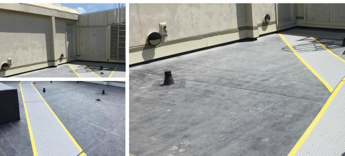
For added assurance, 150mm wide lap tape was imported exclusively for this job (the market norm being just 50mm wide) thus providing 200% greater protection at the seams. 36 substrate vents were also installed, (one for every 50m2) to extract any moisture that may possibly have been in the concrete substrate.
