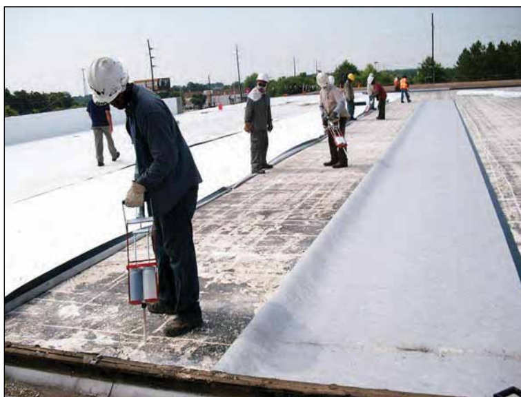
Application of dual cartridges with proprietary caulking gun
