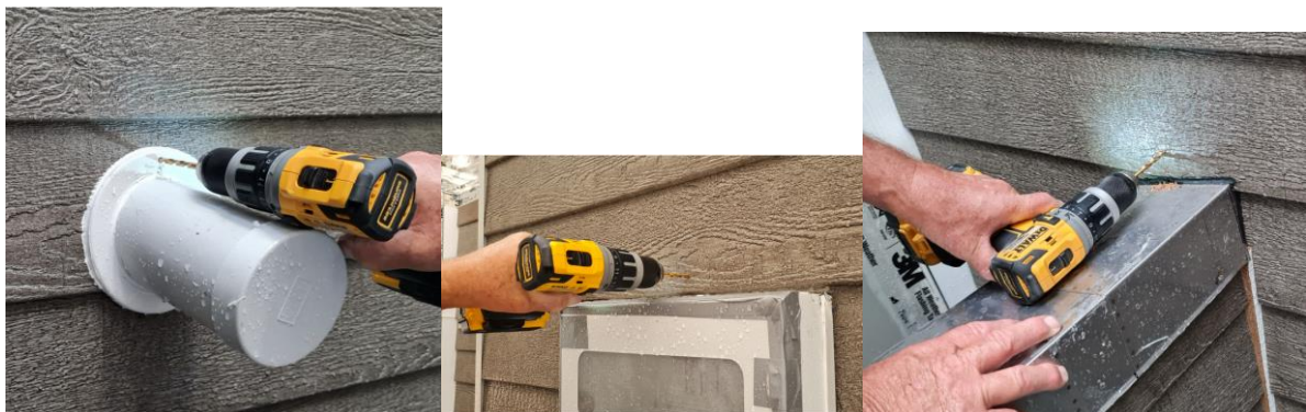
Figure 4: Holes of 6 mm diameter drilled above the pipe penetration, meterbox and balustrade/parapet capping
