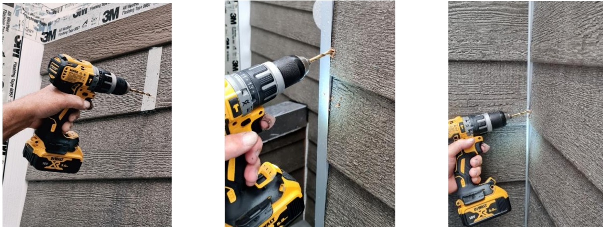
Figure 3: Holes of 6mm diameter drilled in the horizontal jointer, vertical jointer and an internal corner
