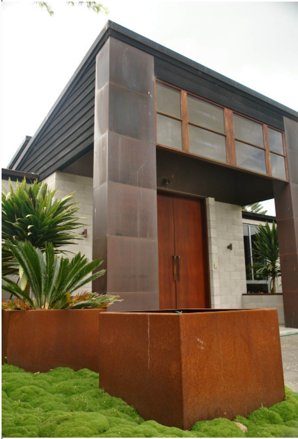
column cladding - copper
