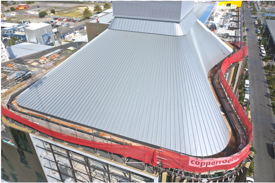
smart tray™ custom roofing - over 900 unique splayed tapered panels with cross welted joints - ARX Aluminium
