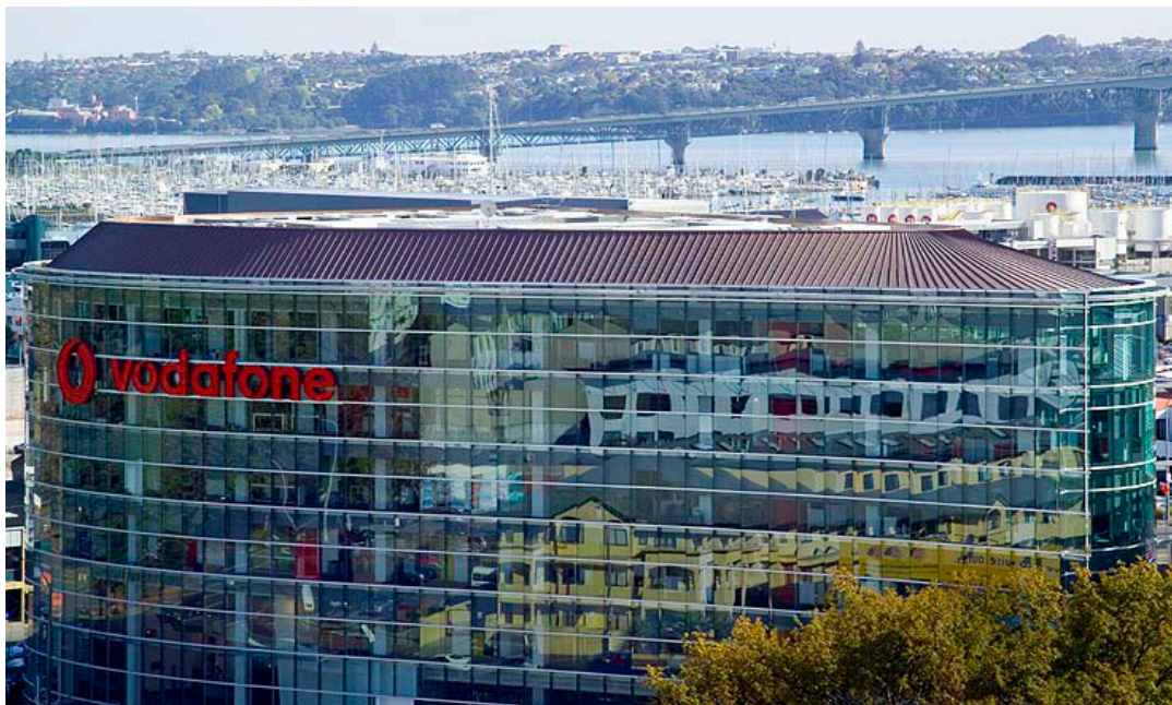
smart tray™ custom panel - splayed copper panels were used to achieve the tight corner radius
