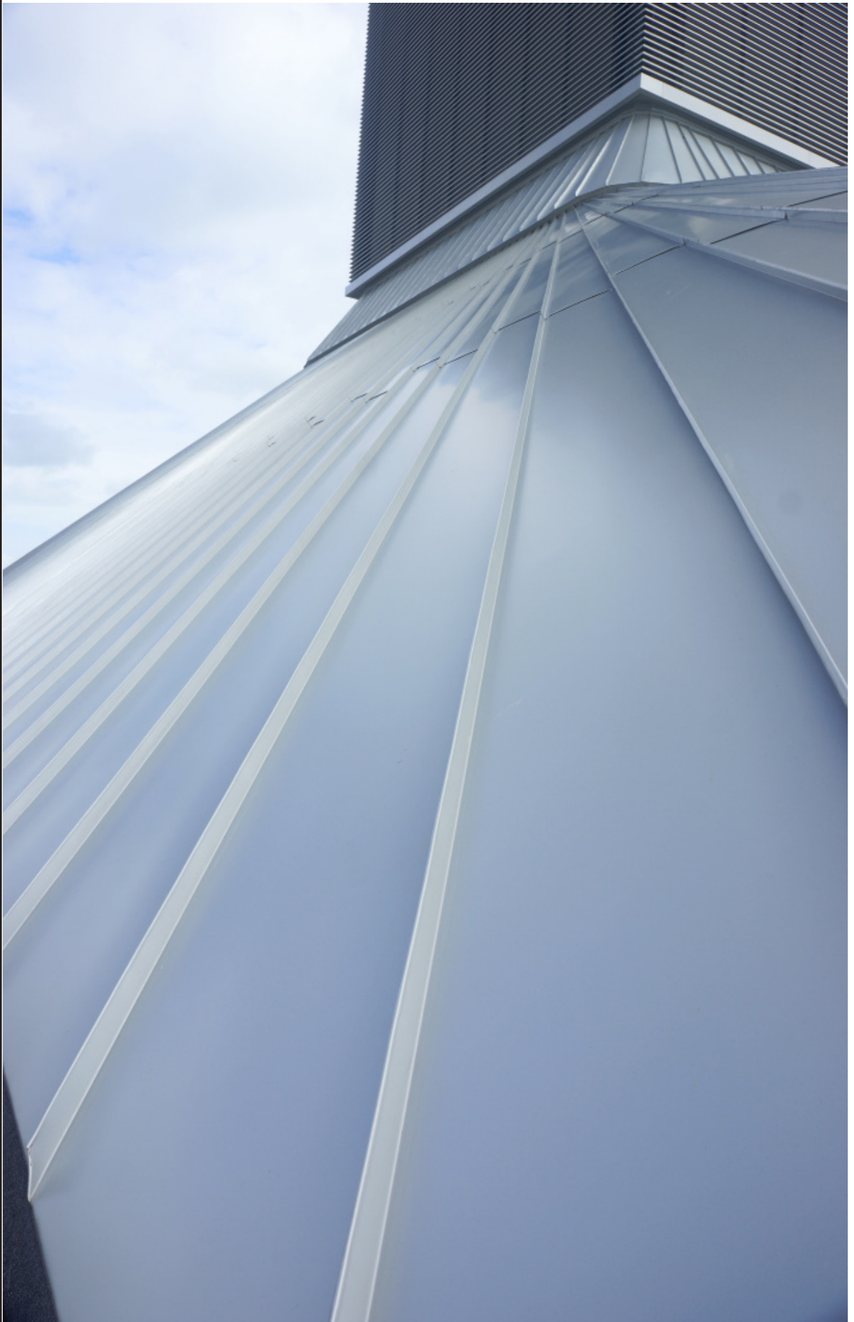
smart tray™ custom panel - tapered aluminium panels created the faceted rolled hips
