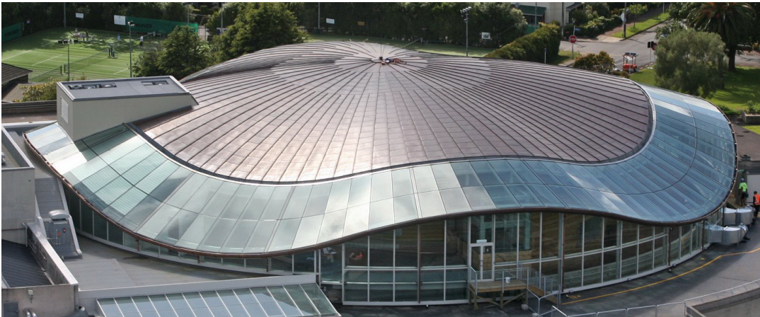
smart tray™ custom roofing - over 900 unique splayed tapered panels with cross welted joints - ARX Aluminium
