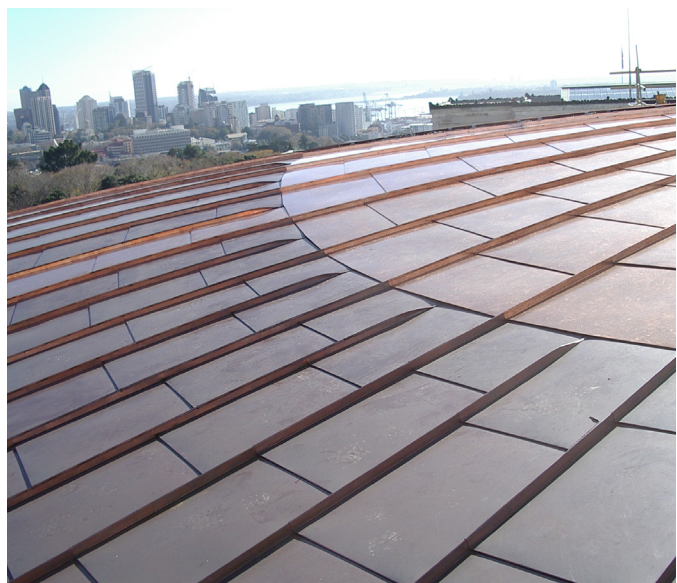
smart tray™ custom roofing - 1760 unique splayed panels with cross welted joints had to be hand folded to accommodate the tapered curved design of the roof - copper
