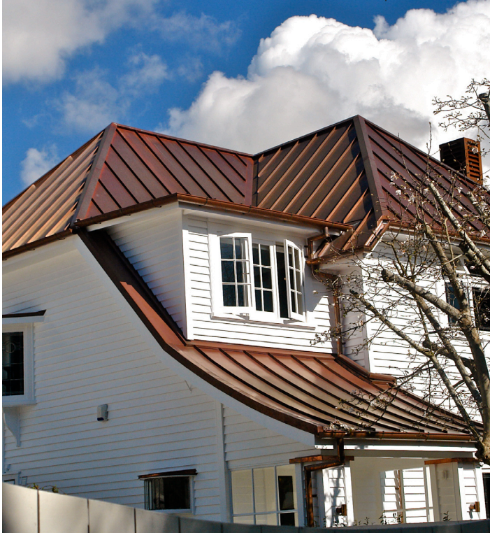
smart tray™ standing seam 38 - copper
