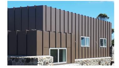
**spanlok**<sup>®</sup> - A revolutionary and recent innovative range of standing seam wide tray roofing and cladding profiles, which have been specifically designed to attach directly to purlins and girts without the need for solid plywood support thereby greatly reducing construction costs.
