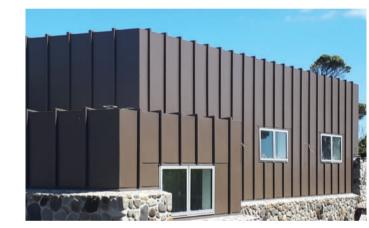
**spanlok**<sup>™</sup> - A revolutionary and recent innovative range of standing seam wide tray roofing and cladding profiles, which have been specifically designed to attach directly to purlins and girts without the need for solid plywood support thereby greatly reducing construction costs.
