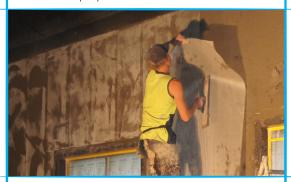
Fibreglass reinforcement application
