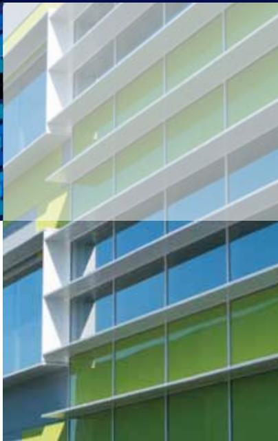
Cleaning should start at the time the products are installed, ensuring that construction materials such as concrete, plaster and paint splashes are removed before they have a chance to dry. Failure to remove these materials at this early stage will require the use of aggressive cleaning materials and techniques with potential damage to the powder coated surface.
