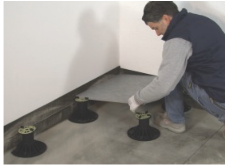
Adjust height with dedicated adjusting key
