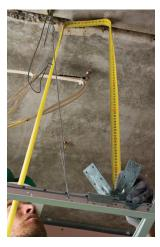
**2/** Measure distance to structure from ceiling grid.
