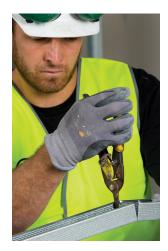
3/ Cut your vertical steel stud to length. Will need to repeat for the two 45° steel studs as per plenum chart provided.
