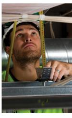
**5/** Measure distance to structure from fly plate below screw holes.
