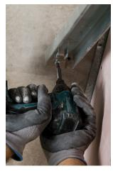
**10/** Fix TRACKLOK® top connectors to structure over with approved anchors.
