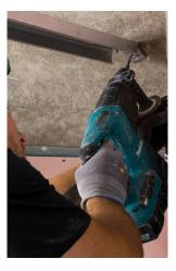
**8/** Drill clearance holes into structure over.
