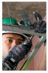
1/ Place GRIDLOK® in position specified on ceiling grid main runner or top cross rail and fix with #10-gauge wafer tek screws.
