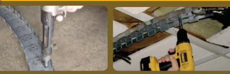
Fasten the track to the ceiling or floor. This secure curve provides for a strong, solid installation.
