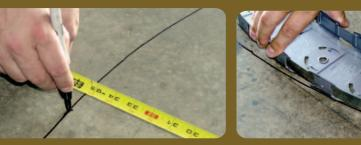
Bend the track to the desired position on a hard surface such as concrete. The pivotal sections of the track make it easy to create the perfect curve with no uneven or flat spots.
