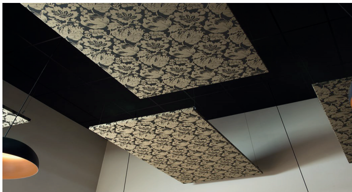
Custom fabric finish suspended on adjustable hangers
