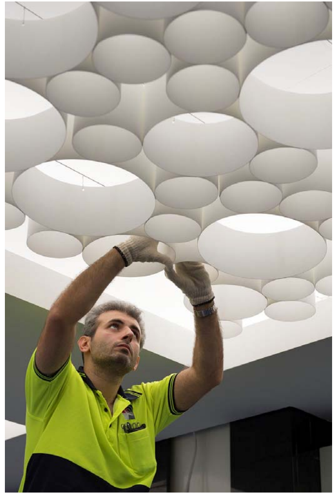
Installation of AO-Gami tubes in ASB Queen Street Branch
