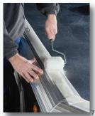
Roll down with a soft roller to conform over contours, seam edges, rivets, or screw heads.
