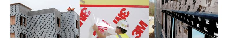
**Non-Permeable Membrane** — Engineered to help control indoor climate by reducing air leakage and uncontrolled airflow through the building envelope and preventing moisture ingress.
