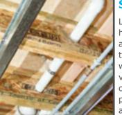
Large diameter holes can be accommodated through the I-Beam web providing versatility and ease of installation for plumbing, ducting and electrical wiring.
