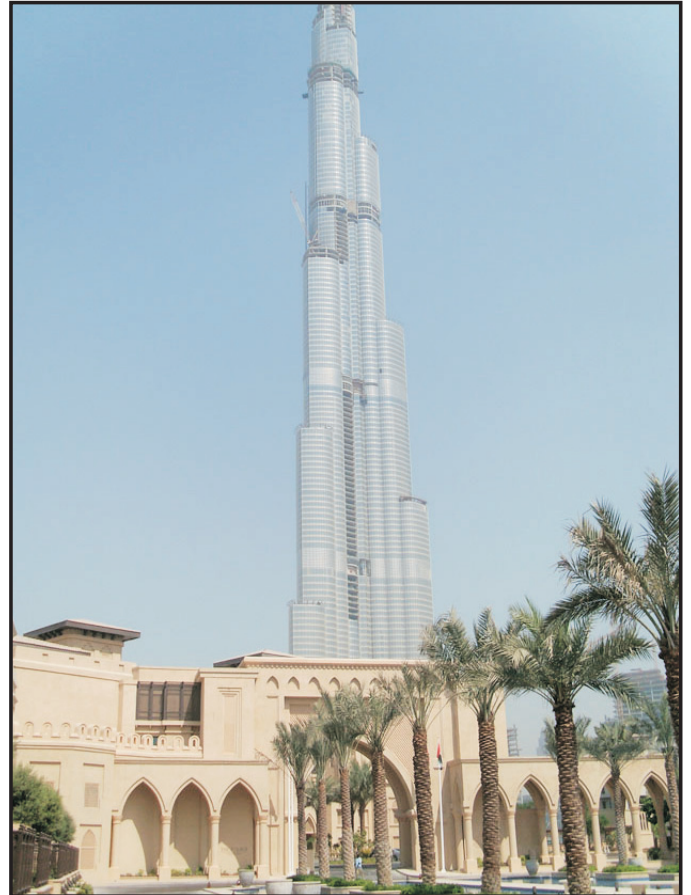
Ecoglo has been recognised as a finalist in the Champion Canterbury Awards because of their innovative approaches and their worldwide reach with product installed in Australasia, North America, Europe, Asia and the Middle East - including the Burj Dubai pictured above.
