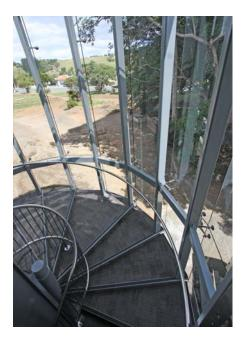
This resulted in a design with 8m high pleated glass hung from the top ring beam with steel clamps. The glass is supported in the centre by stainless steel spider fittings and glazed into a specially designed sill section which incorporated vents to allow air flow into the atrium area. The panels are 12mm grey tint toughened glass with the vertical edges joined together with structural silicon. The effect of the grey tinted glass in the atrium area is stunning.
